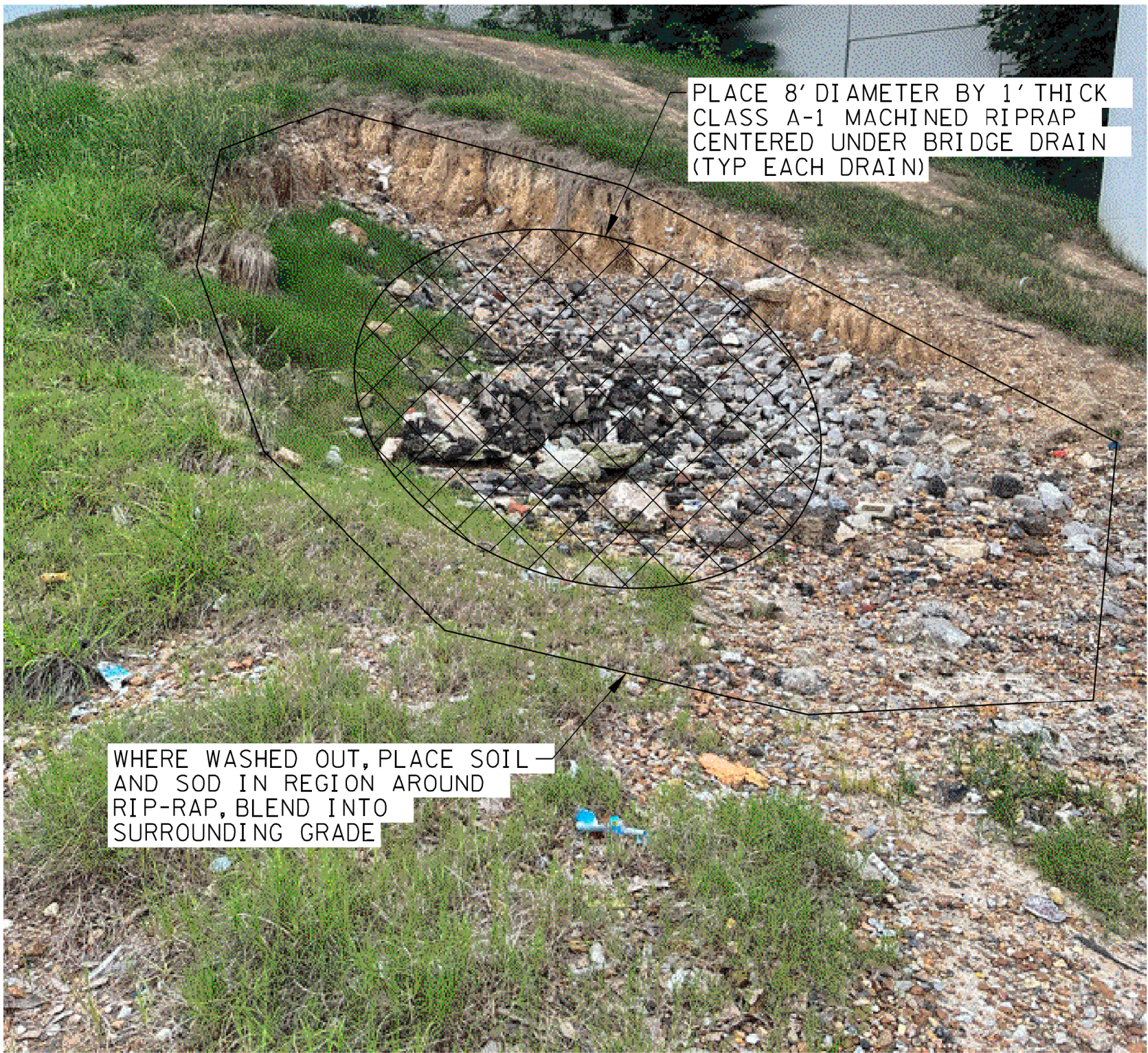
BRIDGE DECK DRAINAGE IMPROVEMENTS (TYPICAL LOCATION SHOWN, OTHER LOCATIONS SIMILAR)
